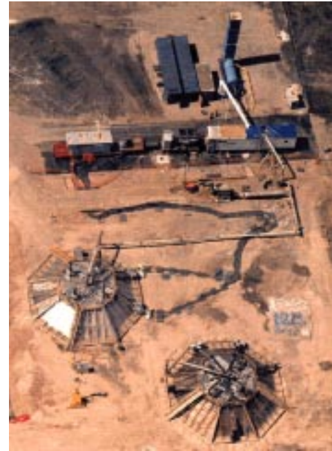
In-situ vitrification hoods.
